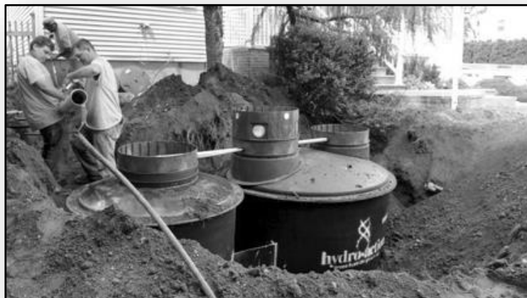
John Crandell and crew from A&A Sewer & Drain install Hydro-Action advanced septic system during Pilot Program
