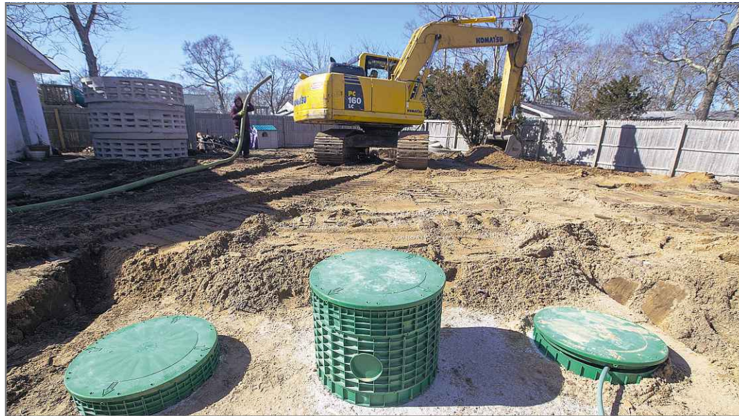
An advanced septic system that removes nitrogen is installed at a home in Flanders on Feb. 27, 2018.
