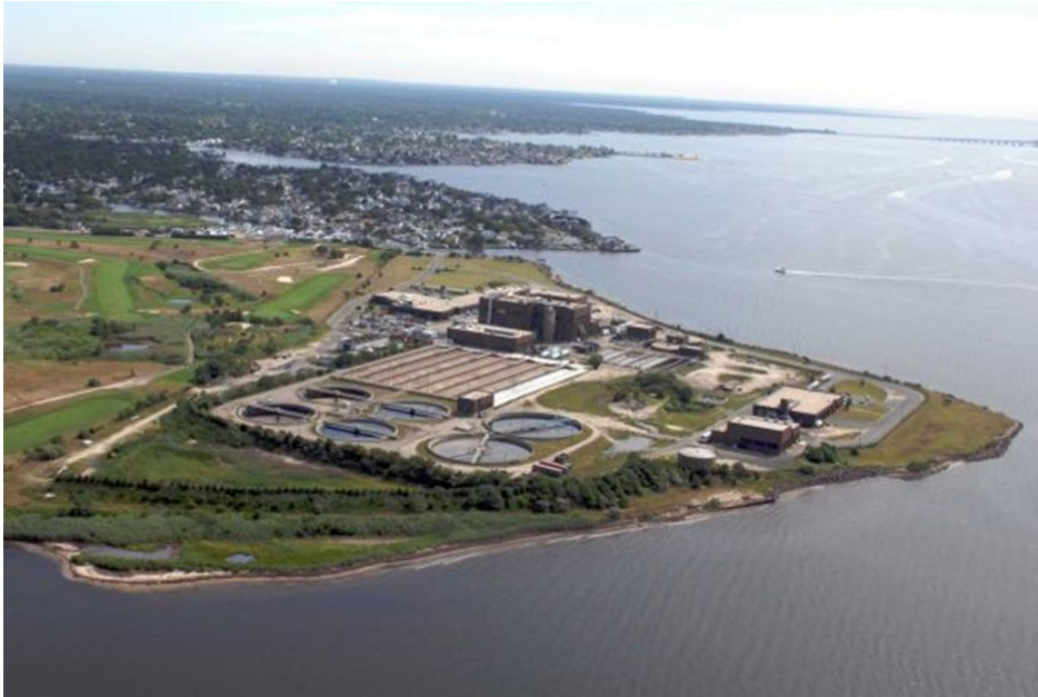
Figure 1-24 Aerial Photo of Bergen Point STP (Courtesy of Newsday)
