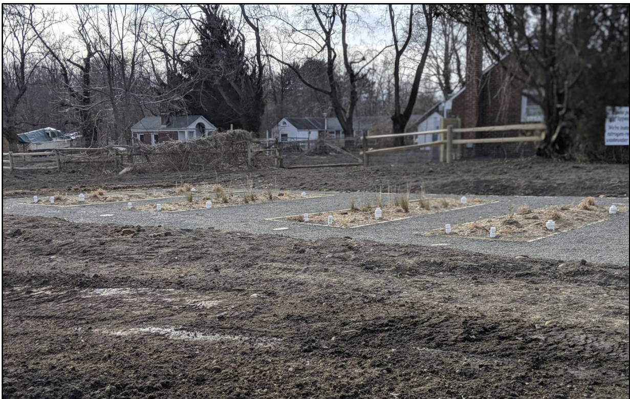
Figure 2-48 Completed Construction of Constructed Wetland at The Nature Conservancy's Upland Farms
