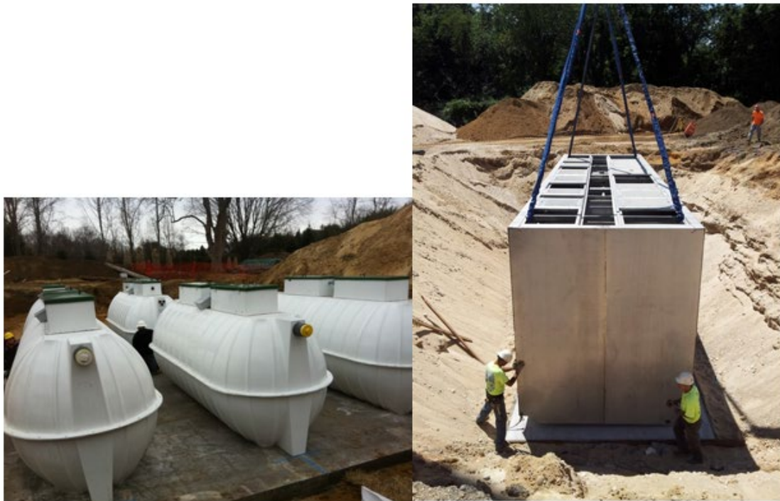
Figure 1-23 CromoFlow (Left) and BESST (Right) Treatment Tanks
