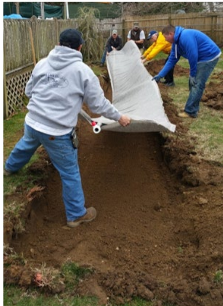
Photo: GeoMat Pressurized Shallow Drainfield Installation
