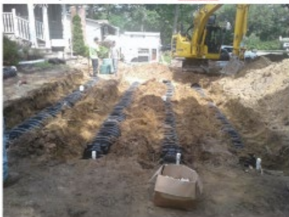
Photo: Infiltrator Pressurized Shallow Drainfield Installation
