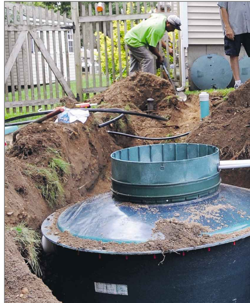
A septic system is installed at a Nesconset home in 2015. About
