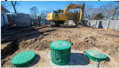
An advanced septic system that removes nitrogen from water is installed at a home in Flanders in 2018. Credit: Randee Daddona
